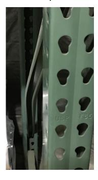
Sure you would detect the damage on the right. But would you have detected the damage on the left?
