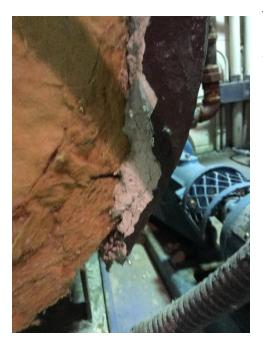
The brown insulation to the left would also be High Damage. Damaged asbestos is clearly exposed and a considerable amount of asbestos is now missing. However, no asbestos debris is present on the floor.
