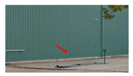
The space between the fresh intake and the exhaust is about 5 feet when it should be 15 – 30 feet.
